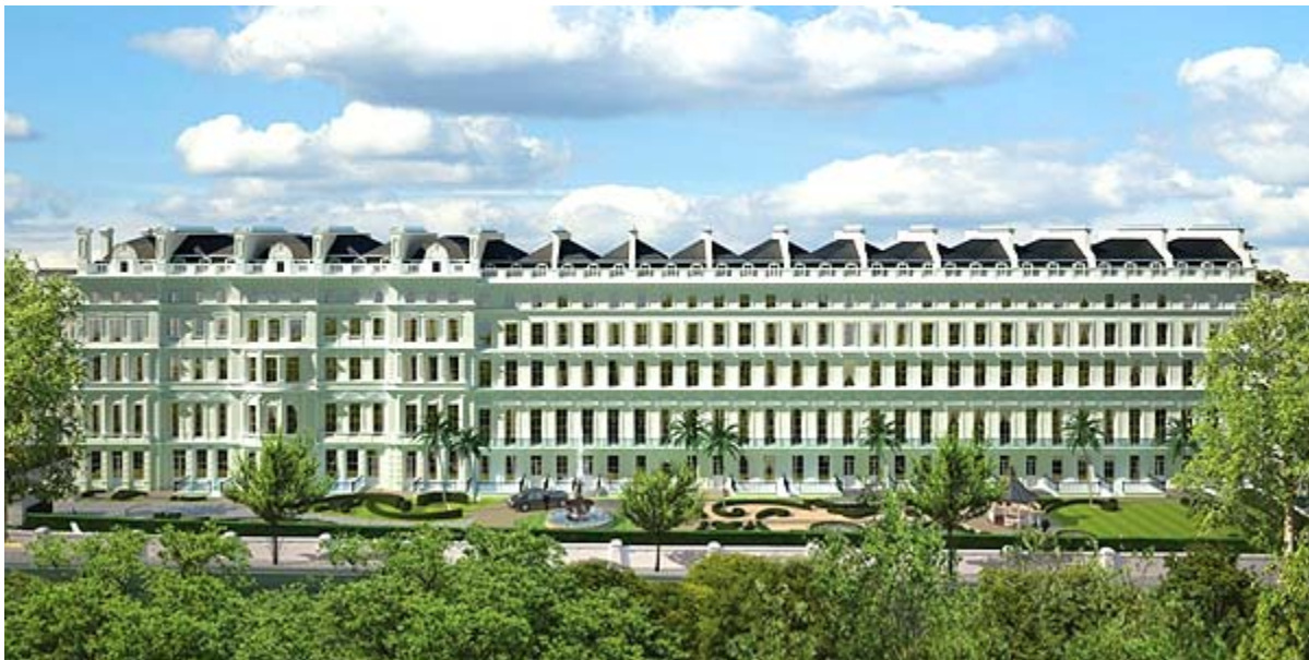
Frontpiece: The Lancasters, a Grade II-listed terrace, in Lancaster Gate, is being converted into apartments
